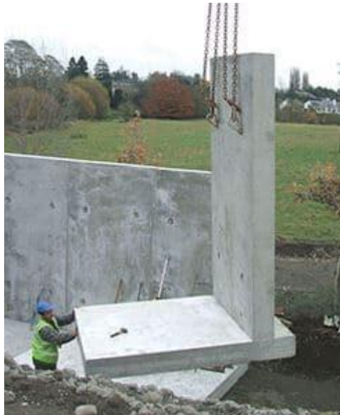
Fig. 1.1. Cantilever retaining wall.
