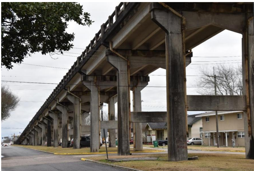
Fig. 5.3. T beam Bridge.
