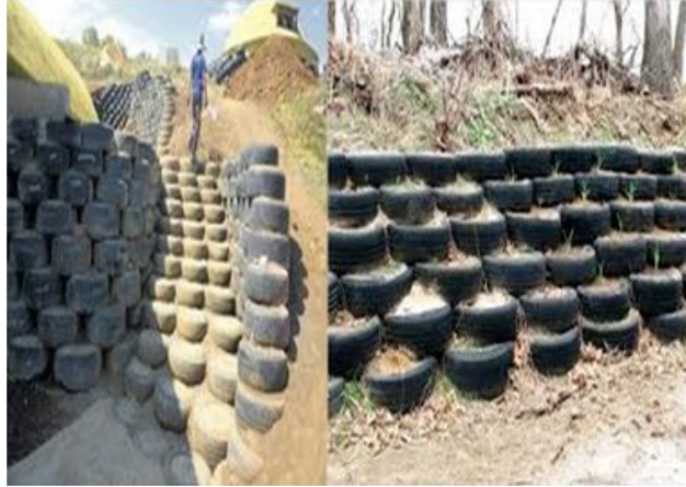
Fig. 4.4: Use of tires as slope-retaining structures.
