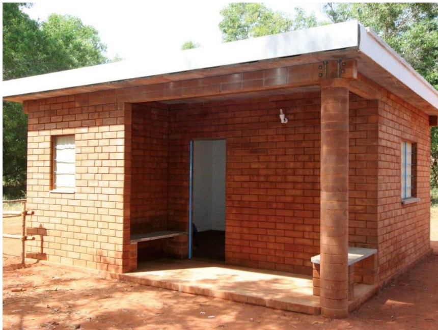
Figure 6.13: compressed earth blocks building
