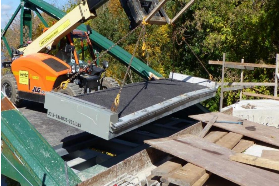
Figure 5.19: The deck slab is made of fiber-reinforced composite panels.
