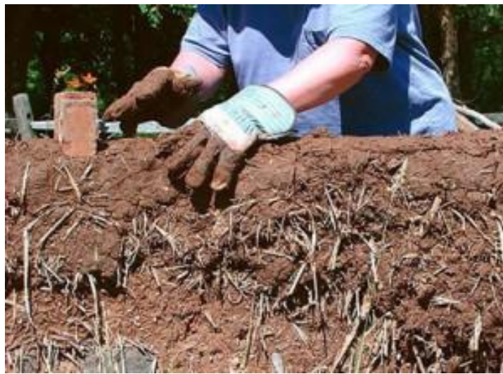
Figure 6.10: COB building technique.
