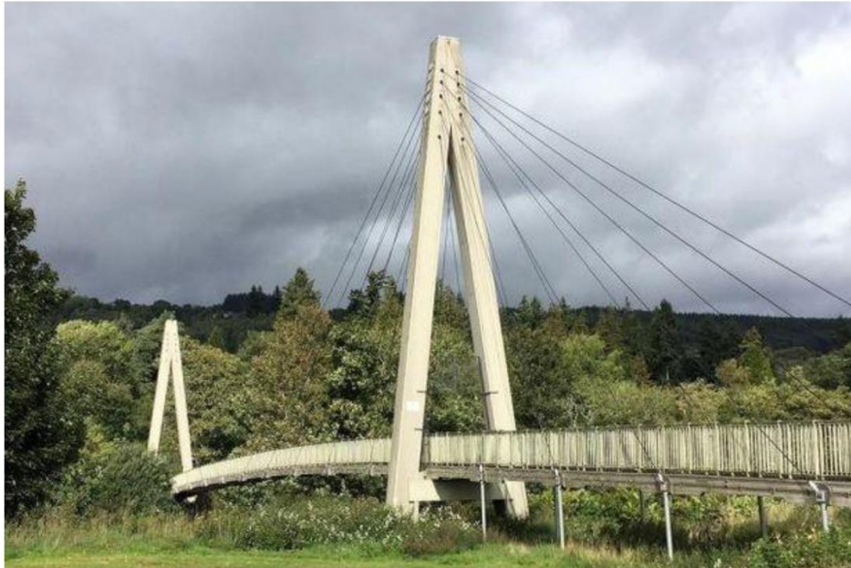
Figure 5.17: Composite cable-stayed bridge
