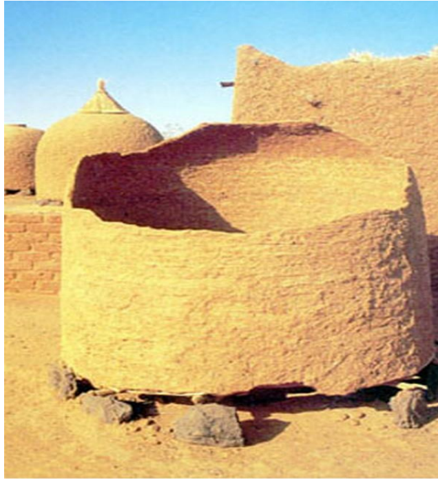
Figure 6.11: Shaped earth building.
