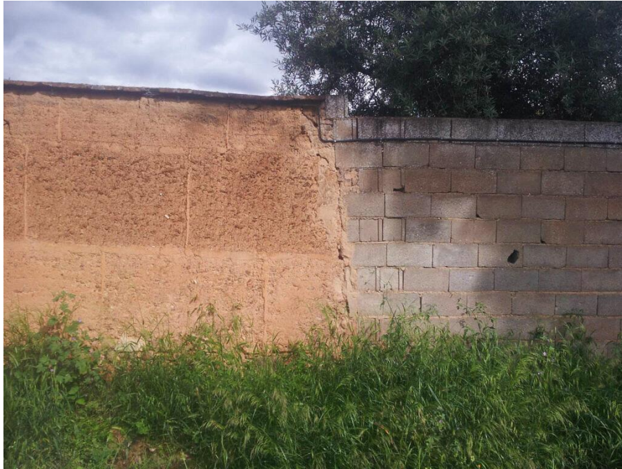
Figure 6.12: Poured earth wall.
