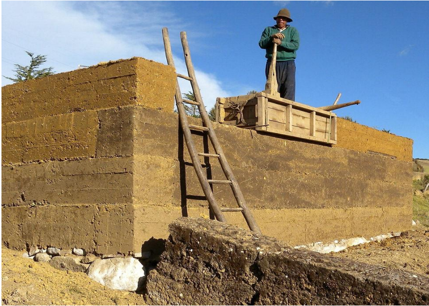
Figure 6.6: Rammed earth construction
