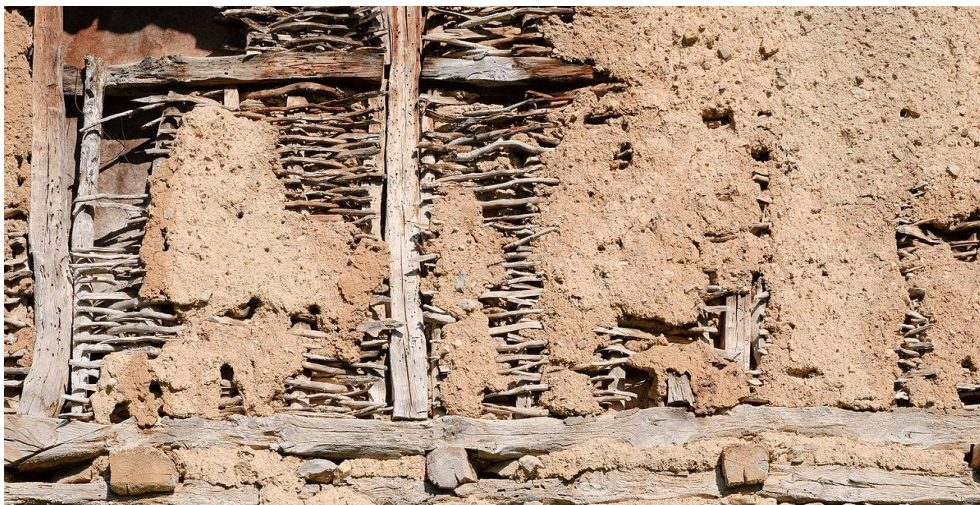
Figure 6.8: Wattle and daub wall
