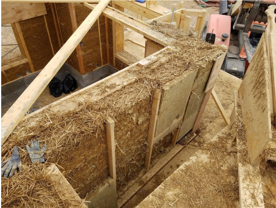
Figure 6.15: Straw clay building process
